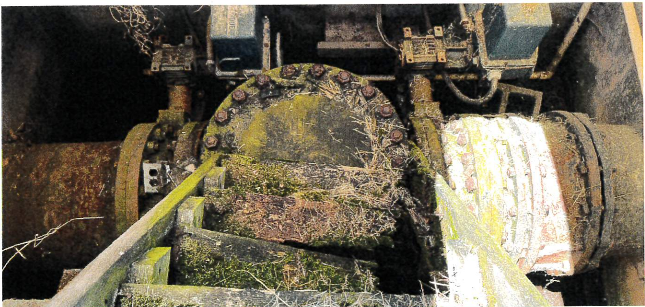
Control valve junction box at plant inlet
